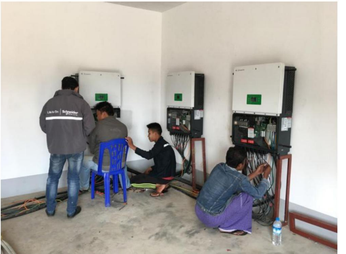
Photo: installation of Schneider CL60E inverters
